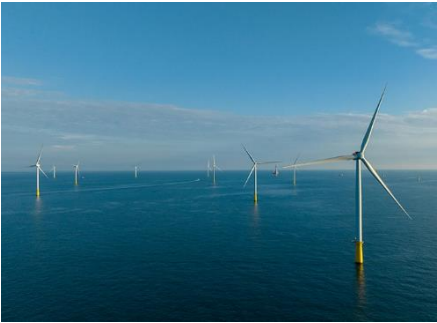
Renewable Energy (Offshore Wind) Business (Taiwan)
